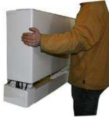
7 Remove the casing.
