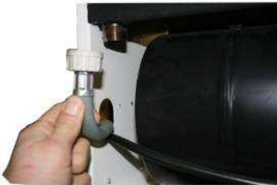
8 Spin condensation pipe.
