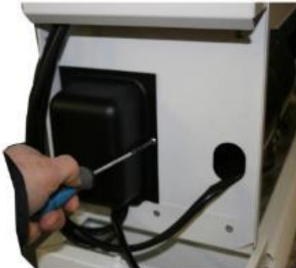
10 Connect power and remote humidostat wires.
